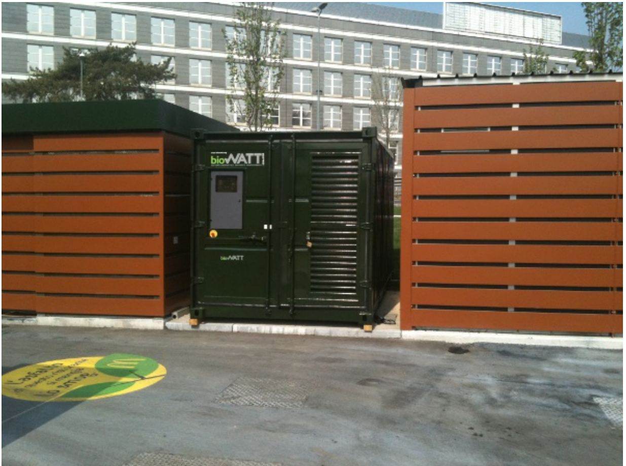
Containers for special wastes, Lainate Restaurant
