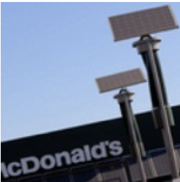
Foto voltaic panels, Lainate restaurant.
