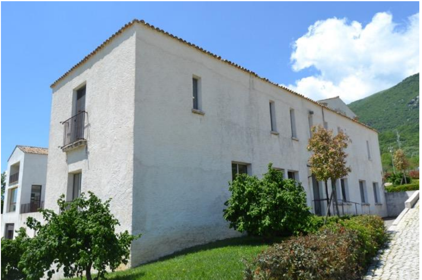
THE SIDE OF CASADONNA WHERE THE SCHOOL IS PLACED
