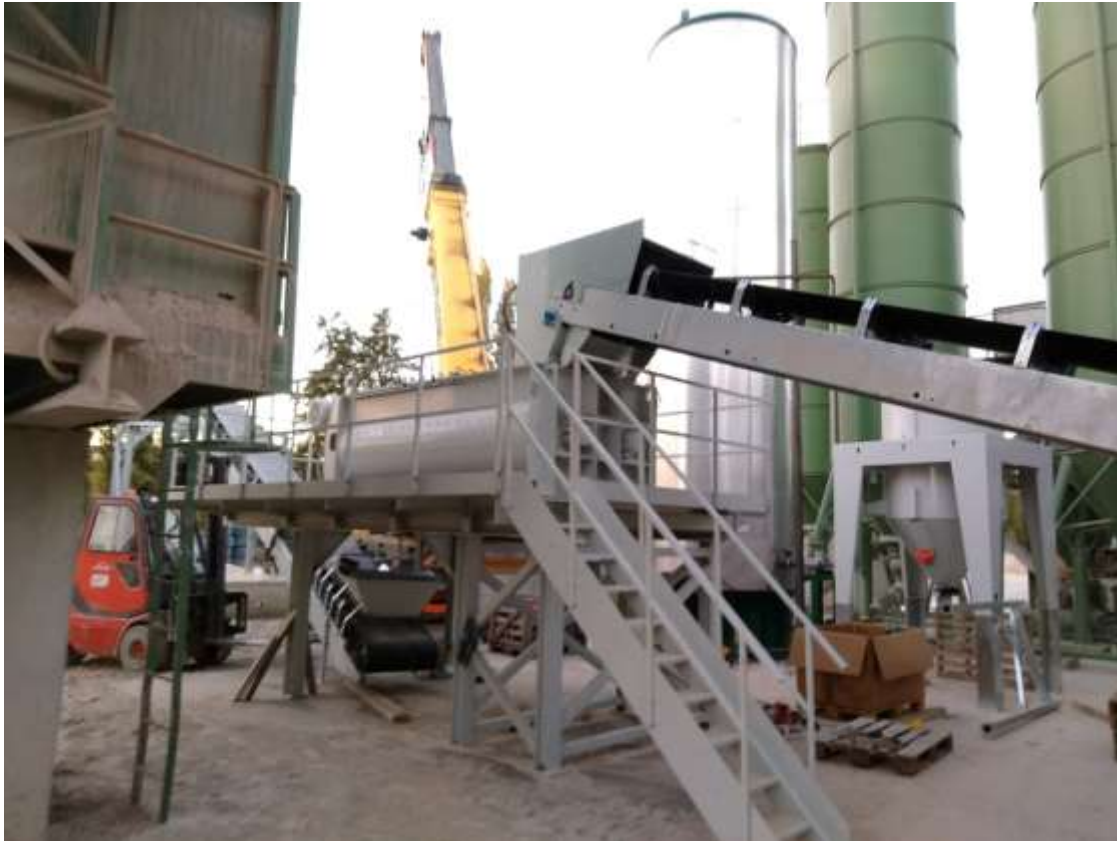
Photo of the plant during the assembly phase
