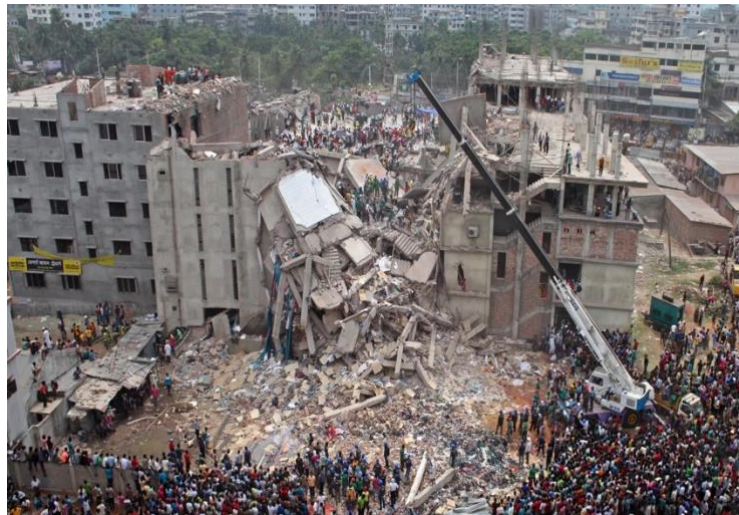
Figura 3: The Rana Plaza building collapse in Bangladesh, April 24, 2013. Photo: Zakir Hossain Chowdhury/Anadolu Agency/Getty Images
