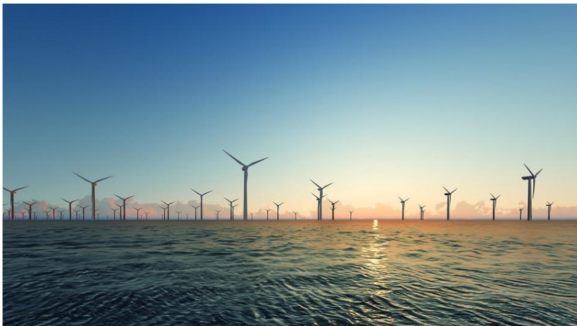
Figure 4: Hornsea Project One, the world's largest offshore wind farm
