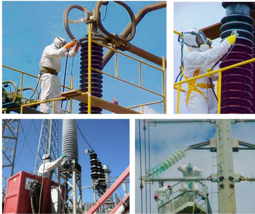
Figure [3]. In-field application on RTV coatings in Brazil (top) and Greece (bottom).
