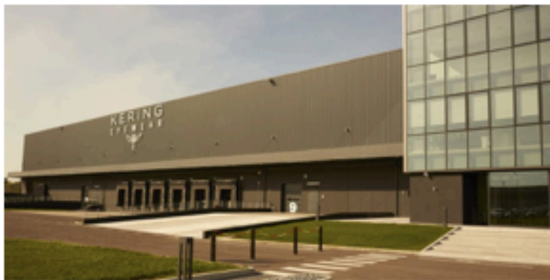
Figure 8 – The Kering Eyewear Logistic HUB (Distribution Center)
