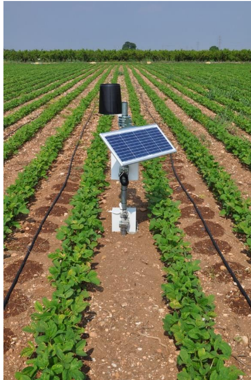
Photo 5: Self-powered irrigation system with photovoltaic panel. Photo Source: Il Nuovo Agricoltore
